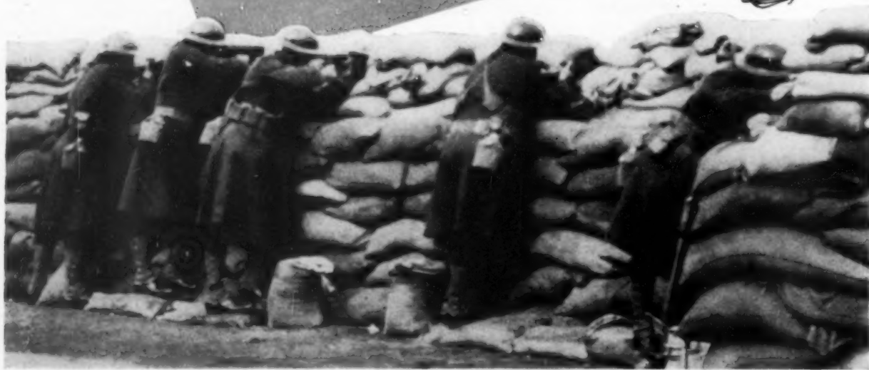
Sandbag emplacements and full battle gear were used by the Fourth Marines during the "thirties."
